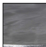
Concrete Steel Base
